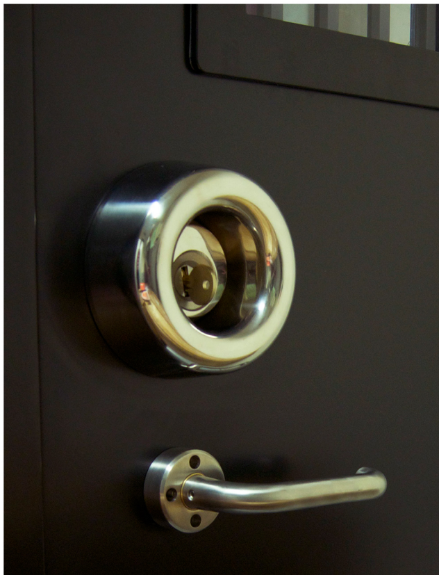
External locking options of lever handle and high security cylinder guard.
