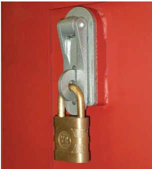
Fire door external locking with Sunray 6000 hasp and staple.
