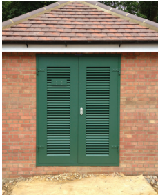
Newly fitted Heavy Duty Doors on transformer building.
