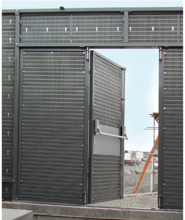
Rear of Louvre Doorset showing panic bar system and anti-vermin mesh.
