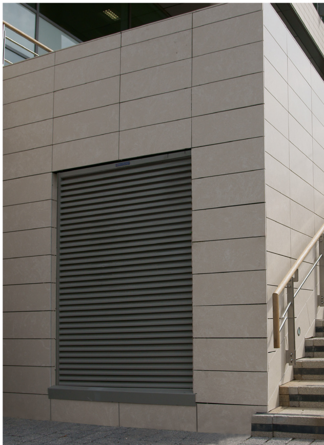
Newly installed Stackable Louvres powder coated in stone grey to blend in with surrounding stone cladding.
