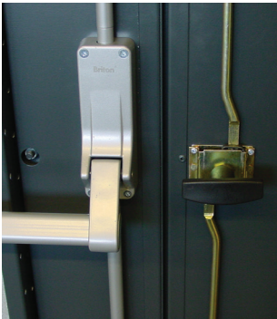
Panic bar and two-way quick release.
